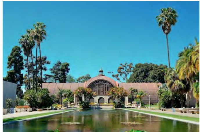
The wood lath Balboa Park Botanical Building, via Freepik.
